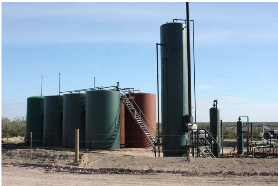
Leighton Oil Storage and Processing Facility
